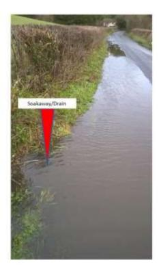
Ponding to half of the width of the lane caused by the blocked drain/soakaway after only a moderate spring rainfall
