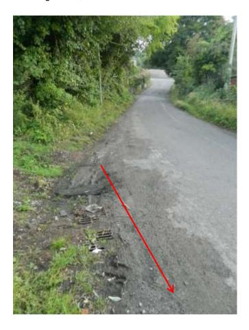
A stream normally flows under the lane left to right where the 2 poles are. Witness marks on the tarmac here opposite the gate to the cricket ground reveal where the over-topped stream and other run-off flowed over and past the drains and on down the lane towards the blocked soakaway (above)
